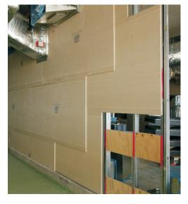
**Easy to Cut & Fix :** FIBEROCK® AT AR Panels can be cut to size by score and snap process using a paper cutting knife.
